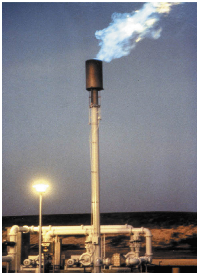
Methane gas flare at a landfill
